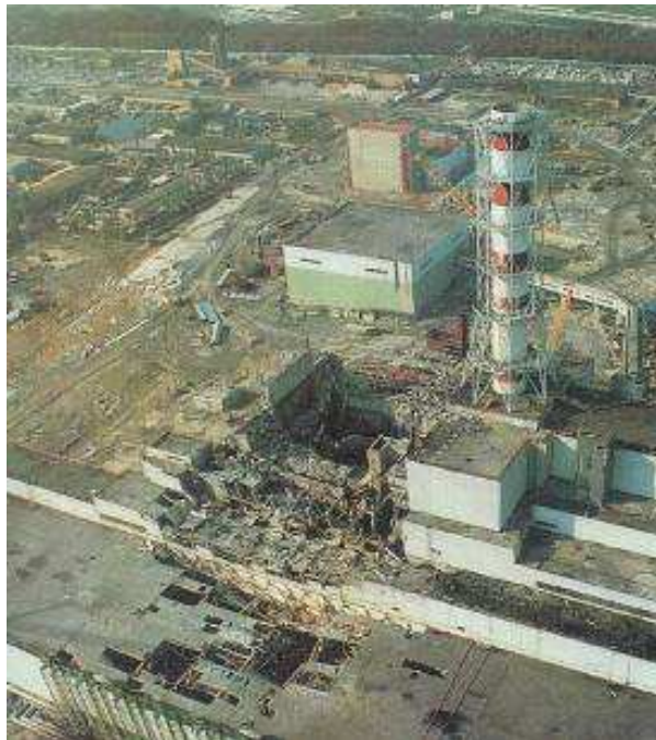
Fig. 4. The hole, the warning, the eloquent and sobering message of a still vivid and silent wound. What remained of Reactor 4 from the Chernobyl (Tchernobyl) nuclear plant in Ukraine (Ukrainia) some time after the explosion, Photo taken in 1986.
