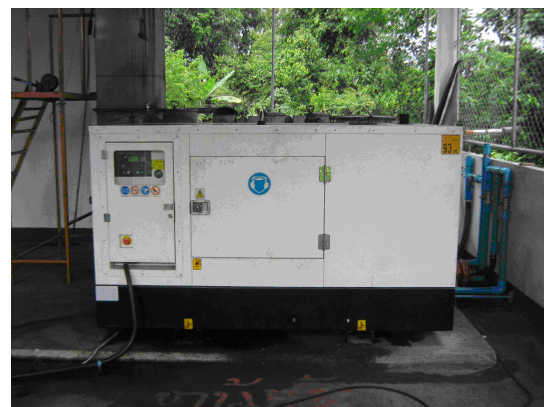
Fig. 4. Electrical generator set.
