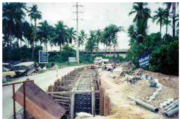
Fig. 7. Open-cut ductbank construction.
