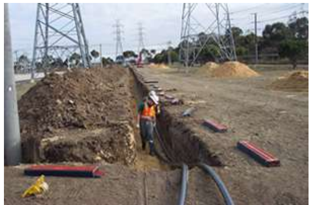
Fig. 5. Direct burial installation [Underground Cable Systems 2010].
