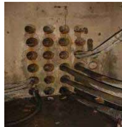
Fig. 6. Cable installed in duct and manhole.
