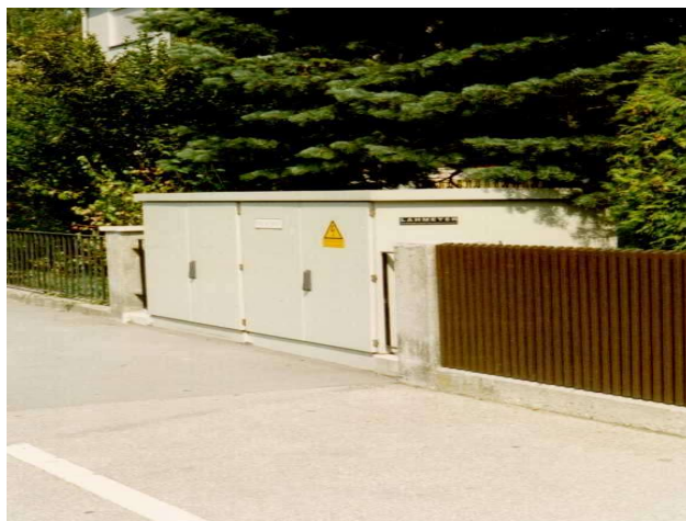
Fig.11. Compact Unit Substation
