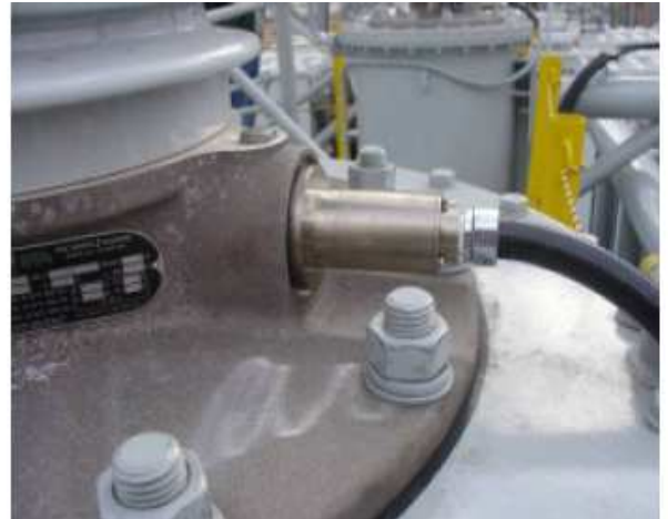
Fig.5. Installed Bushing Sensor.
