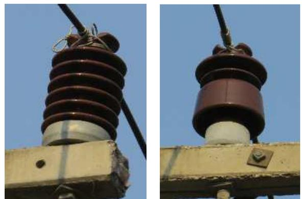
a) Line post Insulator                      b) Pin post Insulator
