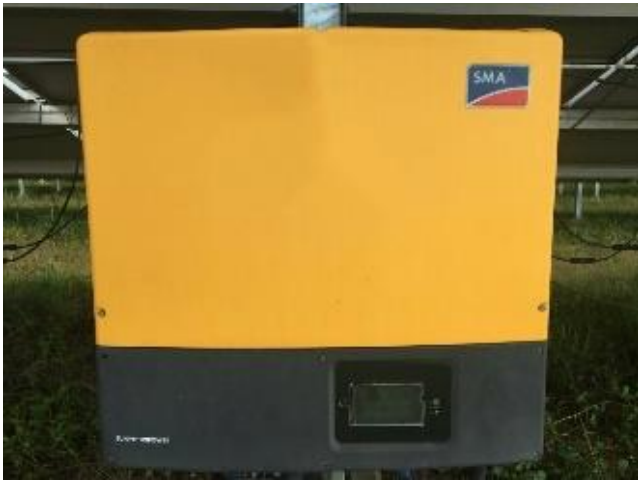
(a) SMA inverter, Sunny Tripower 17000TL model.
