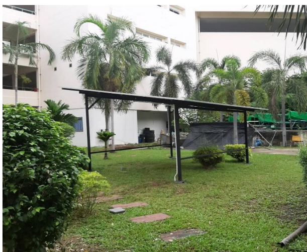
Fig. 4. 3.06 kWp solar cell panels for testing system.
