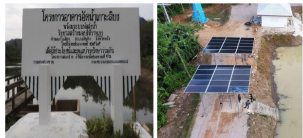
Fig.13. PV of Koh Libong Water Pumping Building Project
